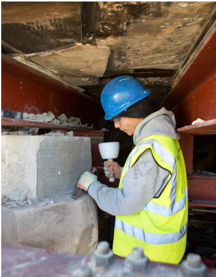
Apprentice carving new stone during the 2015-18 restoration. Copyright © Alan McAteer
