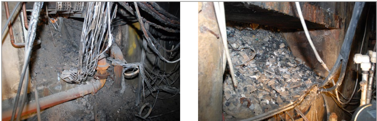
Figure 19 – Cables exiting vertical ducts into level 2 Plenum
