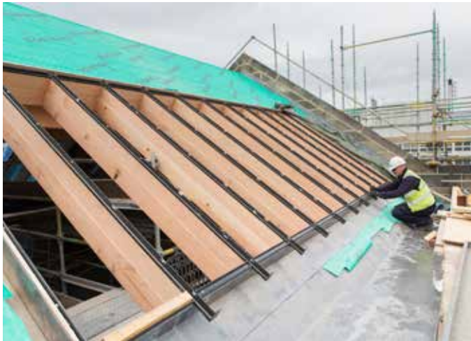
Above: Studio 58 glazed rooflight being fixed in position
