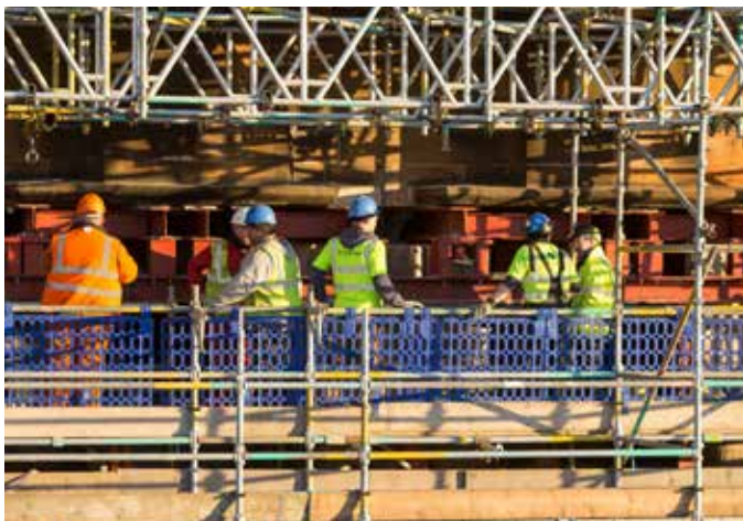
Below: Rebuilding of stonework to library window with temporary steel supports in place
