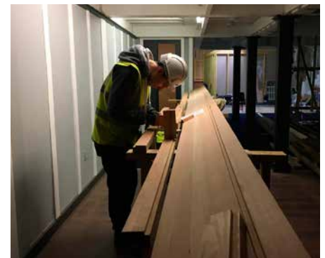
Apprenticeship joiner Reese Cairns, 18, working with WH Kirkwood as part of his 3-year training programme, working on the main screen timbers at The Willow. The project offers tremendous skills-development opportunities.
