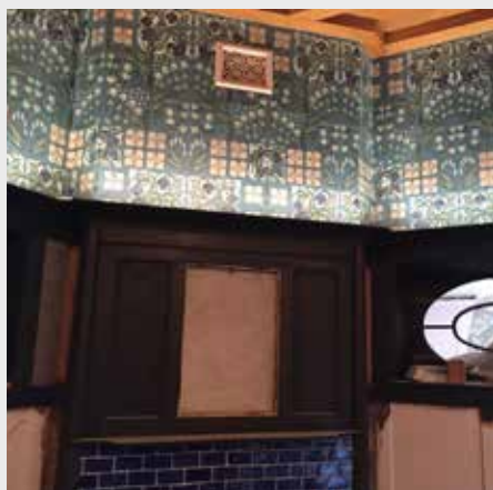
Fig. 7 The original stencilled decoration in the billiards room. This scheme was uncovered and restored by Allardyce and Dundas. This design appears frequently in Walton's interiors. A piece of stencilled linen with the design is in the collection of the V&A.
