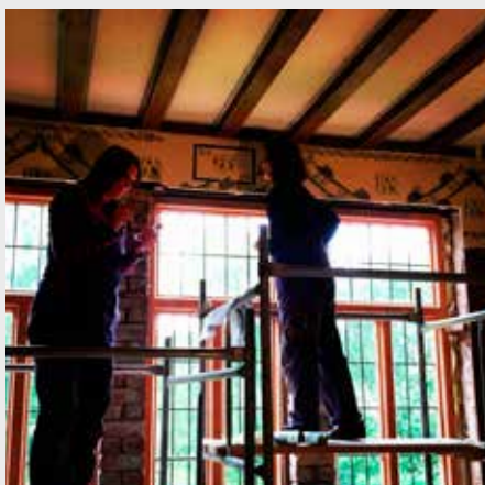
Fig. 8 The entrance hall with the original wood panelling and the stencil scheme restored by Allardyce and Dundas. Metal pieces and glass beads have yet to be added to the blank parts the frieze. This frieze was used by Walton in several properties. At Ault Wharrie he incorporated the initials of the original owner into the design J B S (JB Stewart). Image: © John Cowie
