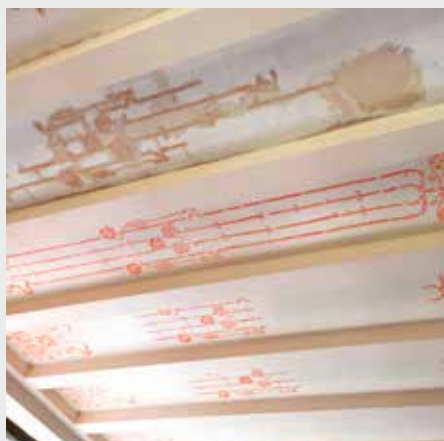
Fig. 10 The sitting room with a stencilled-trellis scheme on 14 ceiling panels between the beams. A small section of the original was recovered from under layers of paint in order to recreate the design.
