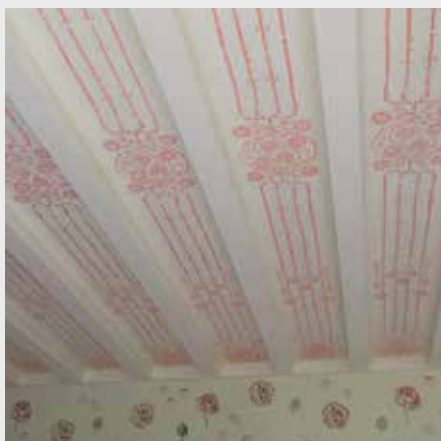
Fig. 11 The completed stencilled restoration in the sitting room by Elisabeth Viguie Culshaw. The original paint was analysed and lecture notes by Walton were referenced to recreate the original.
