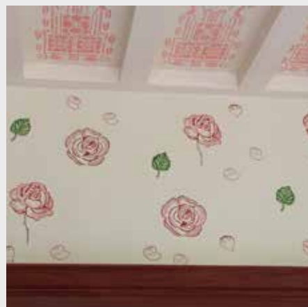
Fig. 12 The rose stencilled border in the sitting room recreated by Elisabeth Viguie Culshaw. Unusually for Walton this design did not have a regimented repeating pattern, but was applied randomly.
