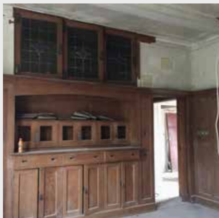
Fig. 4 The oak sideboard in the dining room is integrated into the wall panelling, its upper cupboard still has the original stained glass. This feature is very similar to other properties designed by Walton.
