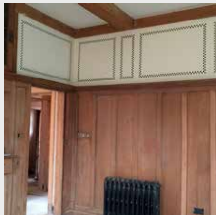
Fig. 6 The restored dining room stencil scheme by Viguie-Culshaw. A photograph of the dining room published in Herman Muthusius's The English House was used to inform the recreated scheme.
