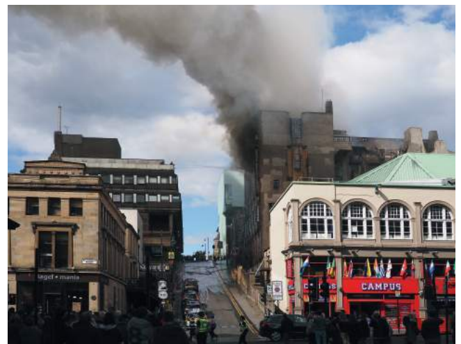
View of the GSA fire from Pitt Street © Stuart Robertson
