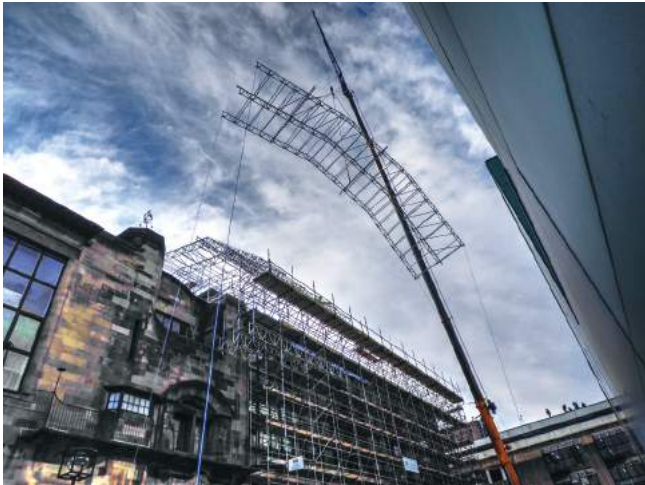
Temporary roof for the Mackintosh Building © Stuart Robertson
