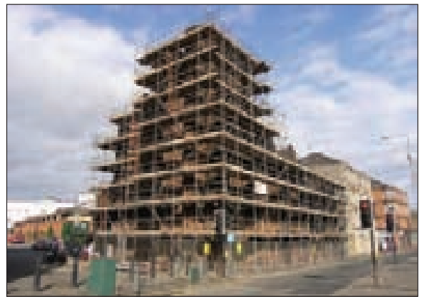
Queen's Cross in 2006 during restoration and refurbishment.
