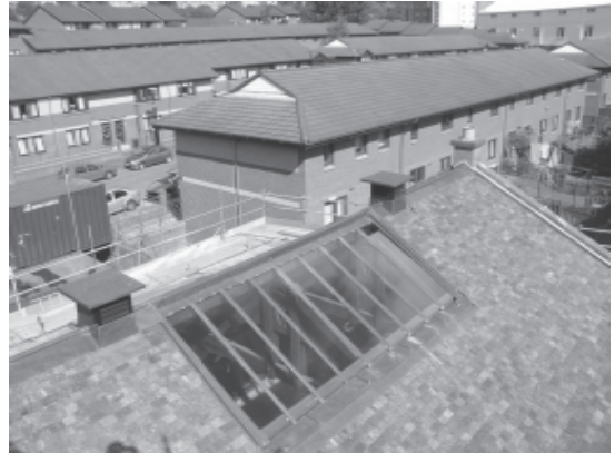
The Hall roof is restored.
